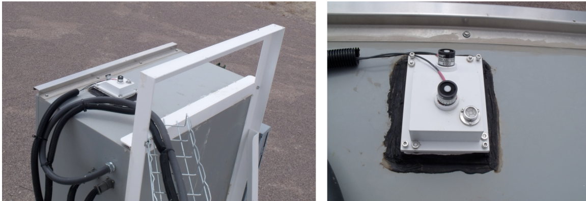
Figure 12. The pyranometers as installed at the VLA site. Pictures courtesy Jerry Langevin.
