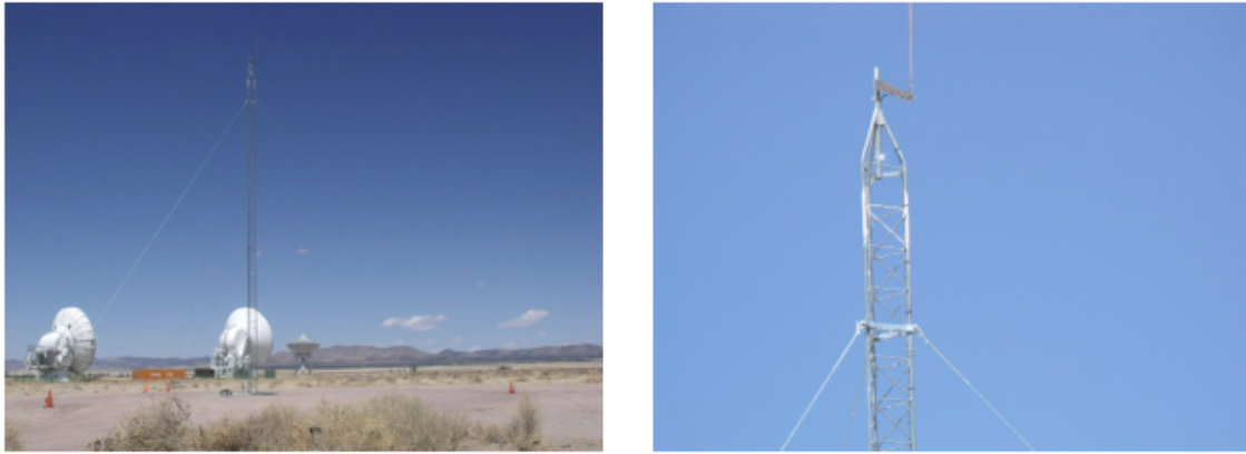
Figure 4. The weather tower, without instrumentation, at the VLA site. On the left is the entire 60' tower (with ALMA ATF antennas and a VLA antenna in the background); on the right is just the top of the tower.
