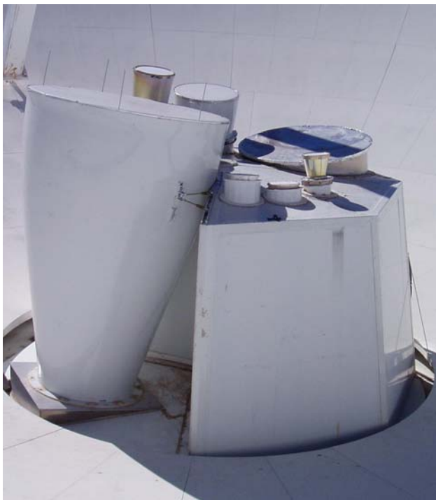
Figure 2 - EVLA Feed Cone Segment
