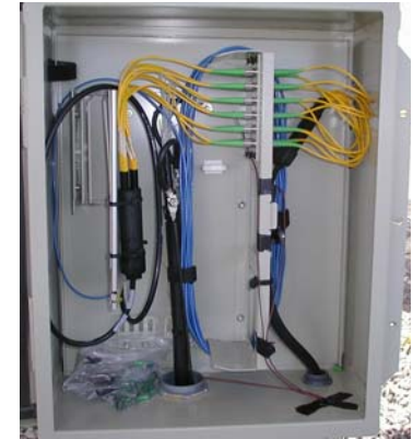
Antenna fiber pad box
