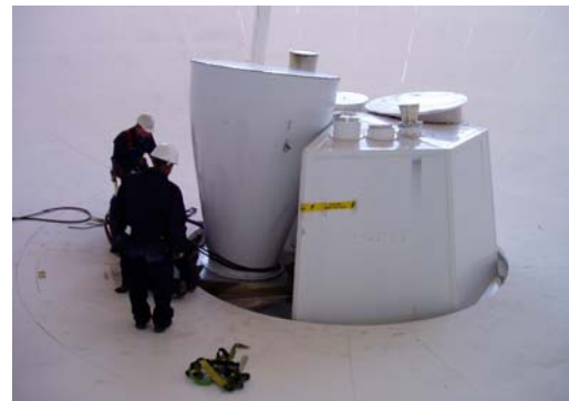
Figure 3b New L-band feed installation on the Test Antenna.
